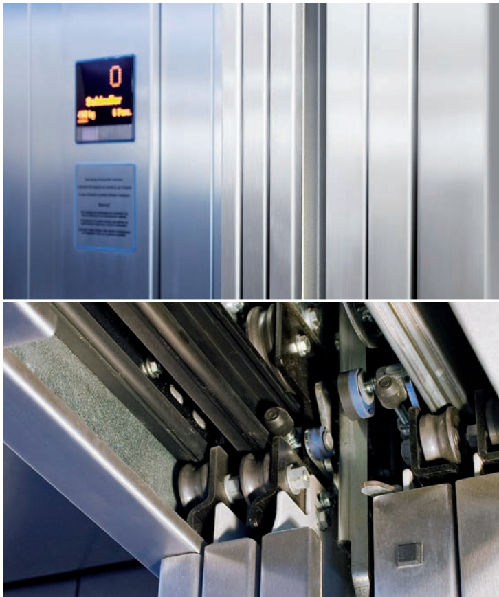
Smooth door operation guaranteed: The long life guide rollers
