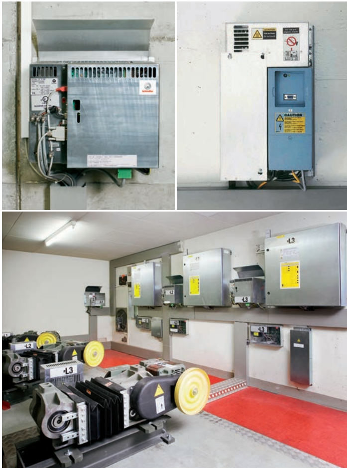
Triplex commercial installation. DR VAB frequency converter linked with a CO MX controller. Powered by DR SGB 142 machine.
