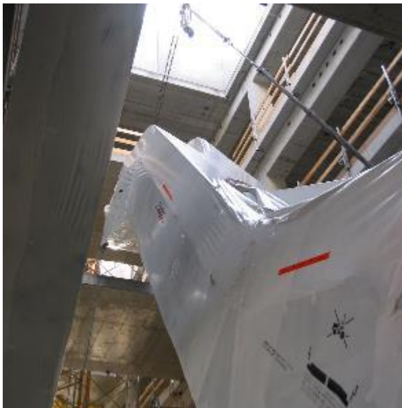
Installation in one complete section by crane
